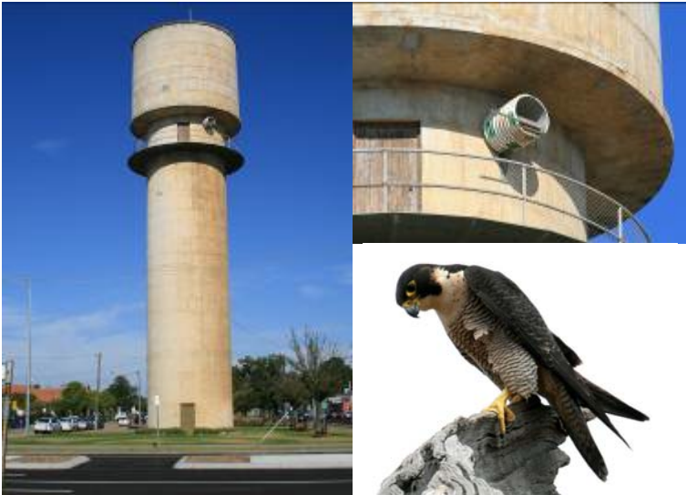
The water tower, nesting box and a potential nester (photo courtesy of Rohan Bilney)
