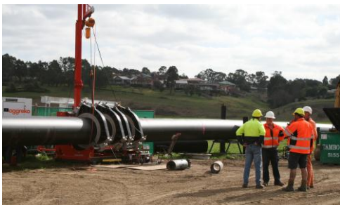
Preparing the replacement pipeline
