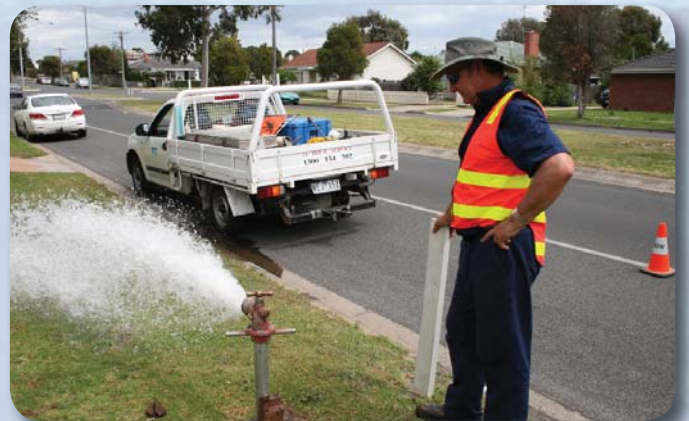
Ongoing initiatives include high-pressure cleaning water mains to keep on top of water quality
