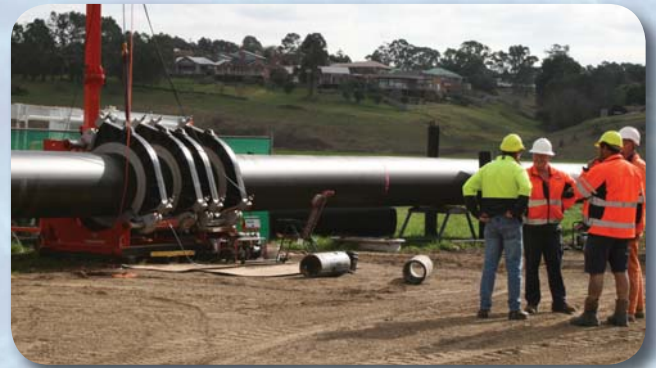
Preparing the replacement pipeline
