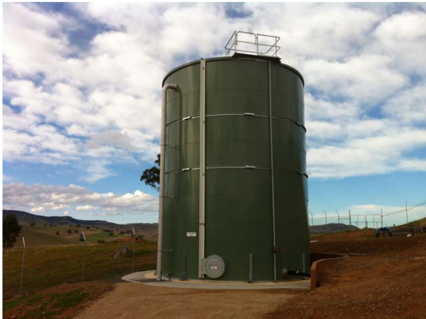
Figure 3: Swifts Creek Tank
