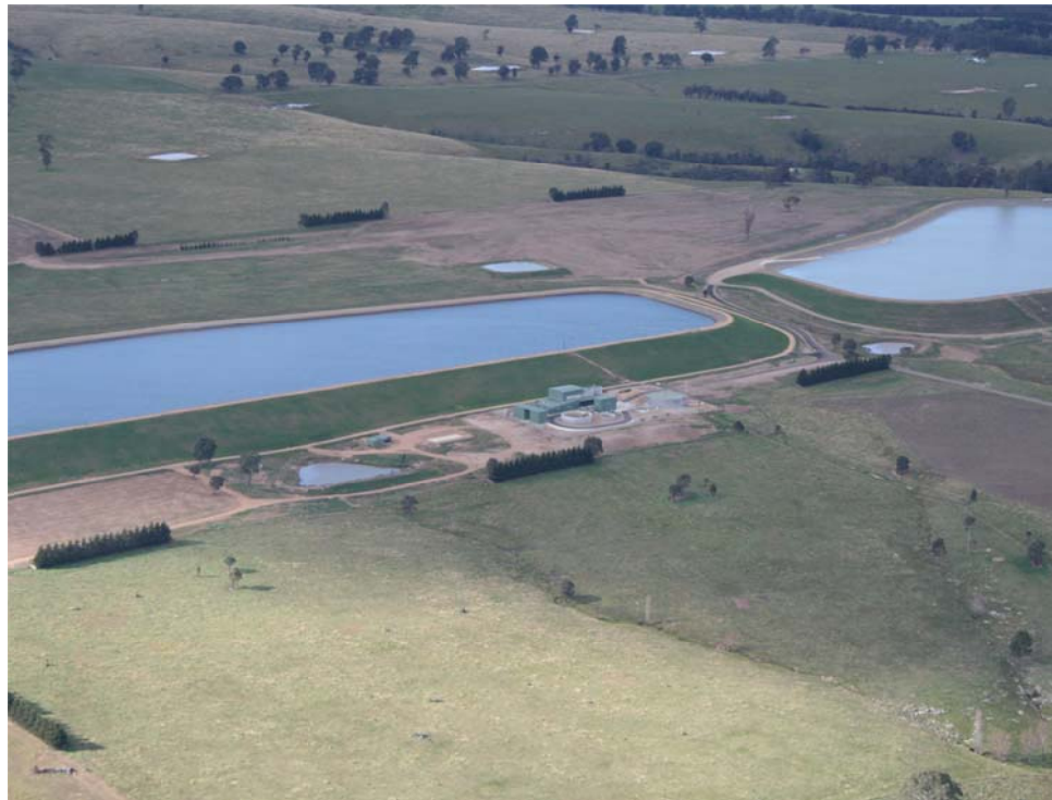
Figure 3: Woodglen water treatment plant and additional raw water storage (right) commissioned in 2010
