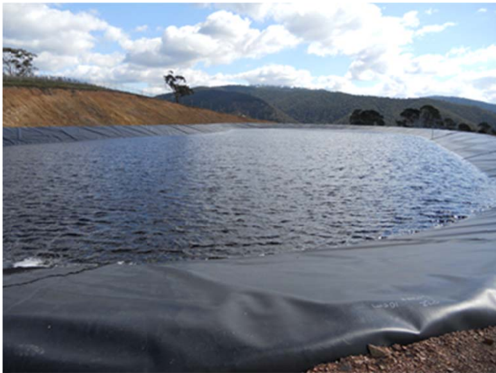
Figure 5: new 10ML raw water storage will ensure the continued quality and security of water supply for Omeo into the future.
