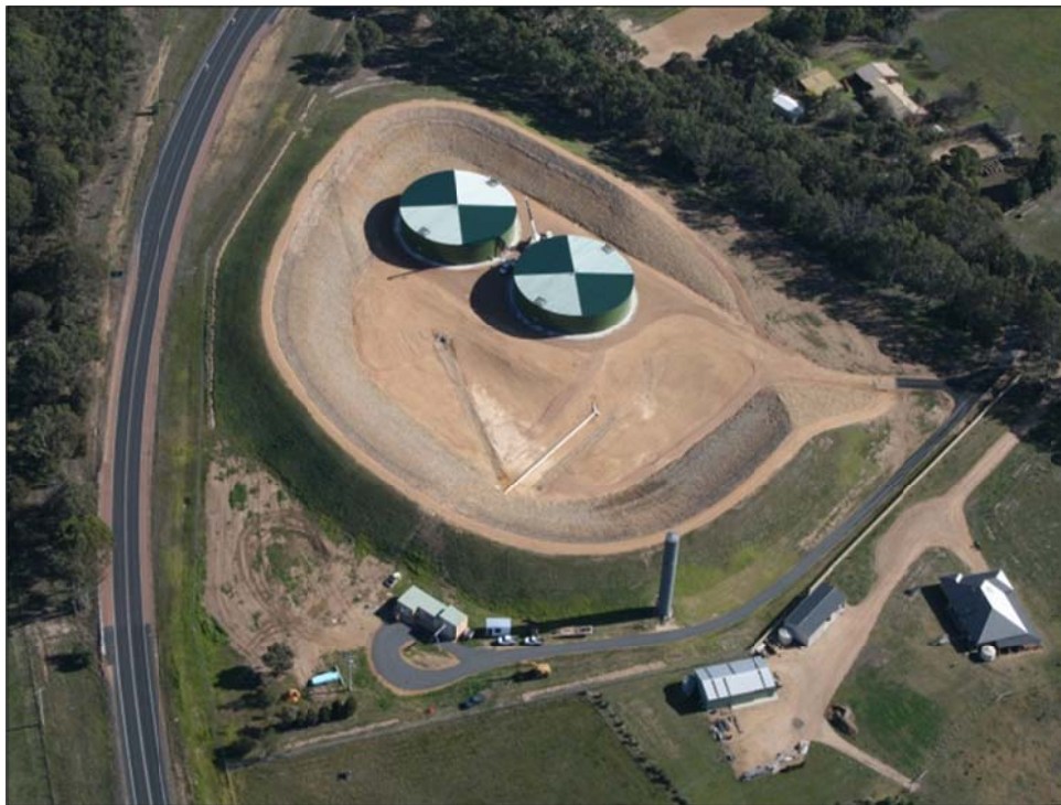
Figure 4: Tanks with 12ML storage capacity replaced an open treated water basin at Eagle Point
