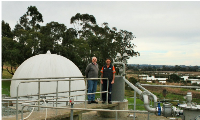
Monitoring the new facility are East Gippsland Water Project Engineer, Hardy Fandrich (left) and Wastewater Treatment Operator, Dino Giove
