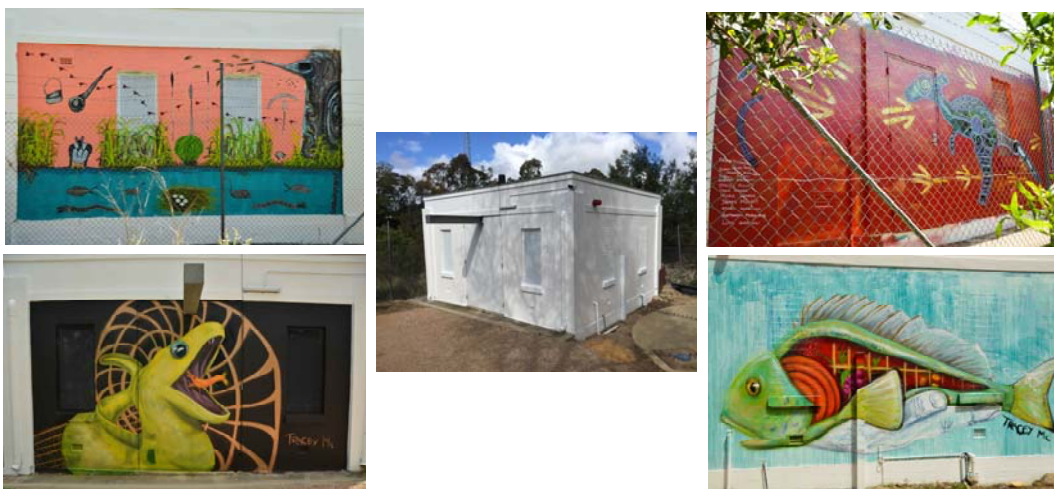
A burst of aboriginal-inspired art brings vibrancy to the once bland pump station building!
