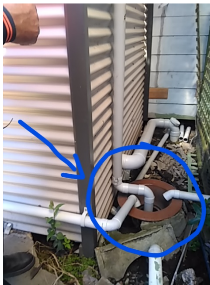
Examples of stormwater pipes illegally connected to the sewer
