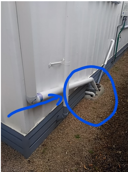
Examples of stormwater pipes illegally connected to the sewer
