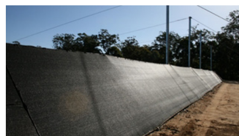
Shadecloth over Mallacoota’s raw water basin
