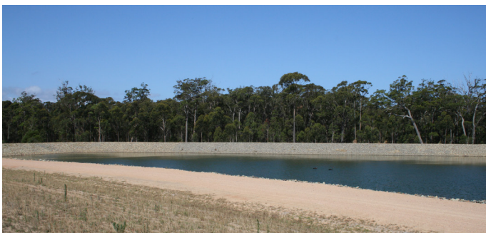
Mallacoota Wastewater Treatment Plant
