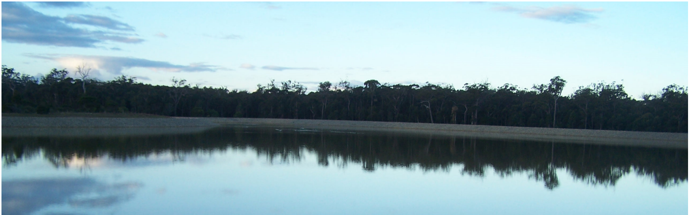
The winter storage basin at the Mallacoota Wastewater Treatment Plant
