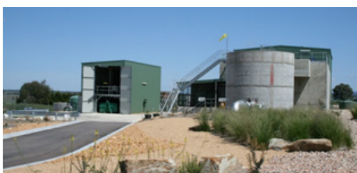
The Woodglen Water Treatment Plant
