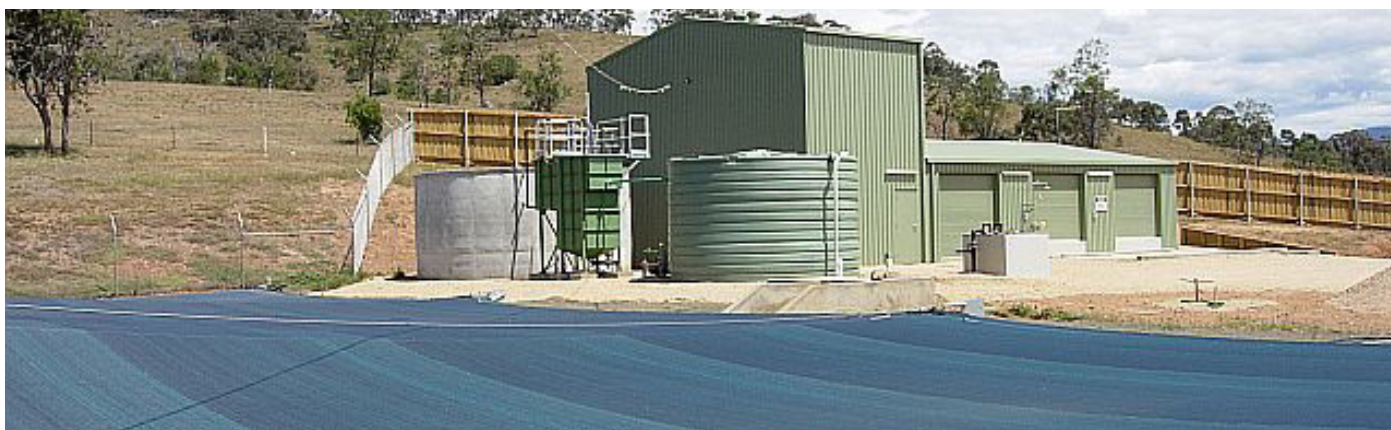
Swifts Creek Water Treatment & Raw/Clear Water Storage (shadecloth on)
