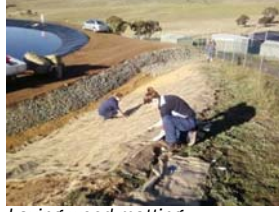
Laying weed matting
