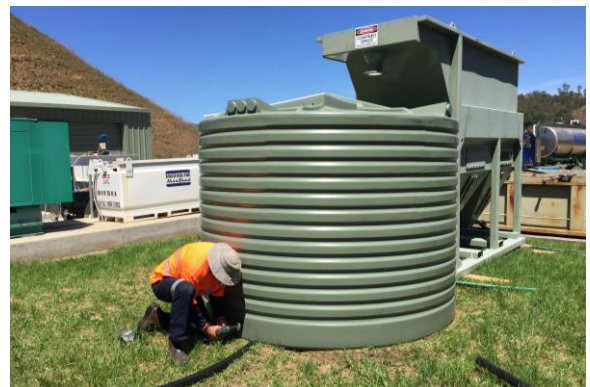
Setting up the portable clarifier equipment to clean muddy Buchan River water prior to treatment
