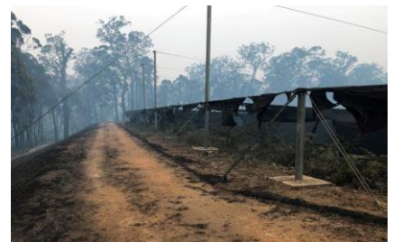
One of the Mallacoota water storage covers badly damaged by the bushfires at the very end of 2019
