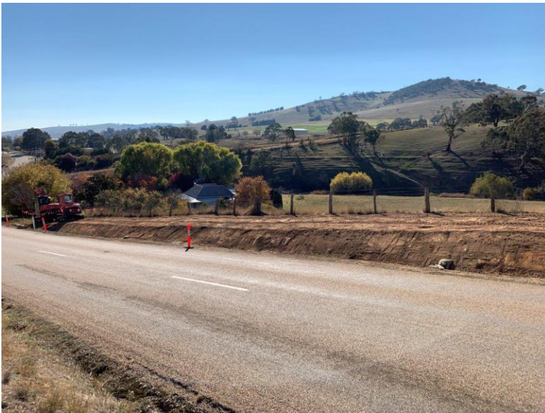
Photo: Work starting on the Day Avenue water main upgrade
