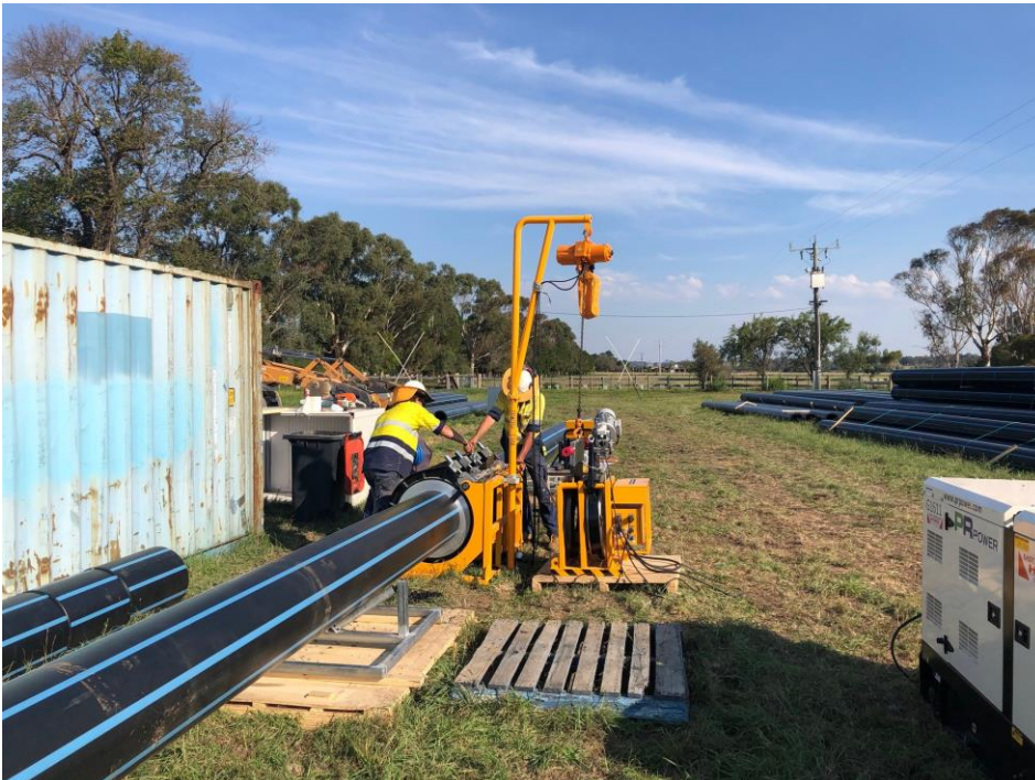
Photo: Work on the Bairnsdale – Eagle Point pipeline
