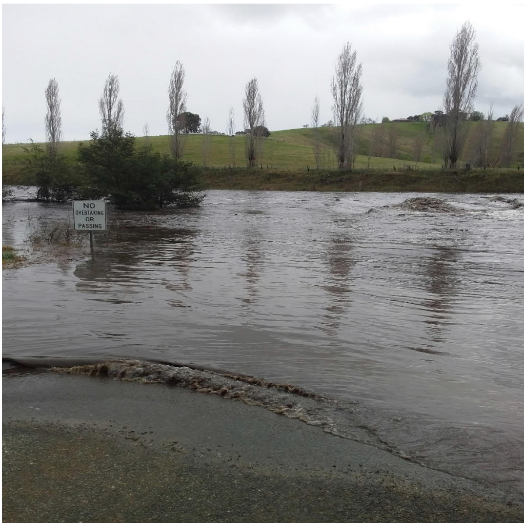
Photo: Old Coach Road Bridge over the Tambo River 15/9/2021.
