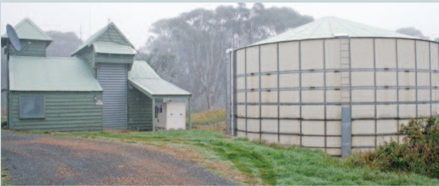
Dinner Plain, showing the storage tank for harvested groundwater
