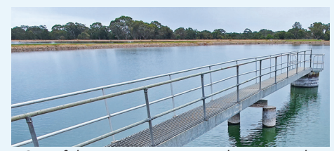
One of the wastewater storage lagoons at the Paynesville wastewater treatment facility
