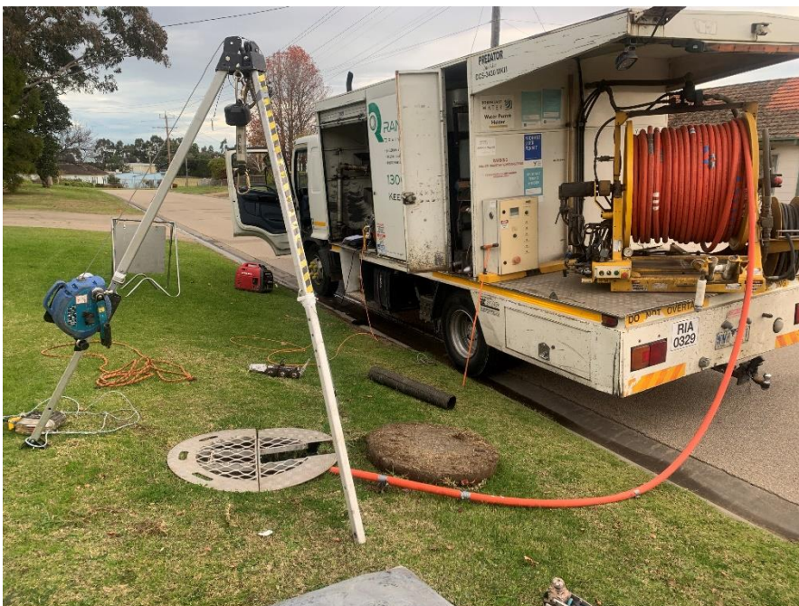
Image: Sewer relining works underway in Bairnsdale.
