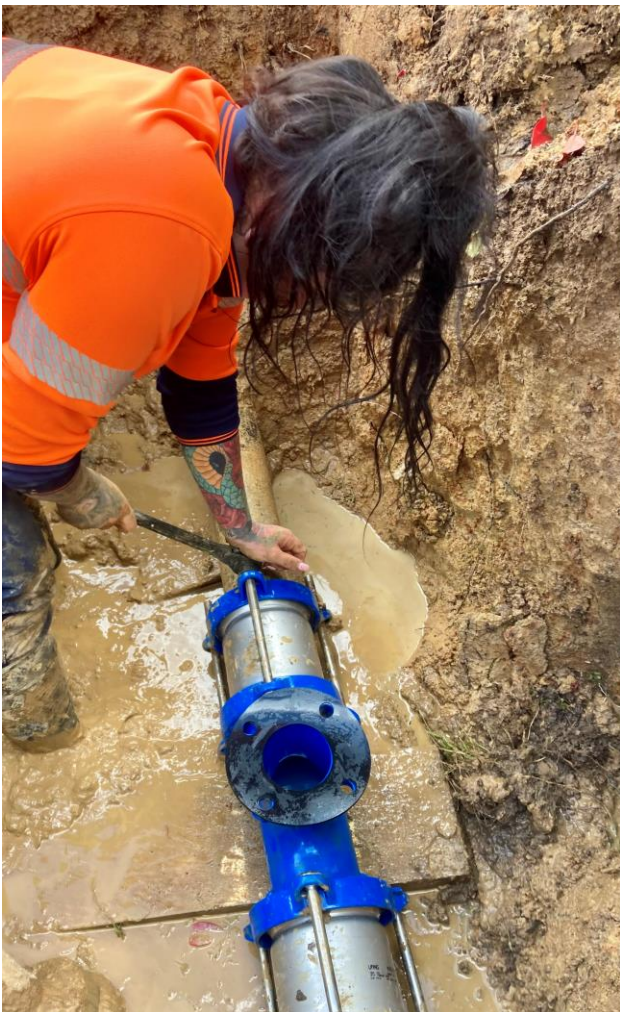
Caption: Gini Eynstone in the thick of it, repairing a water leak.
