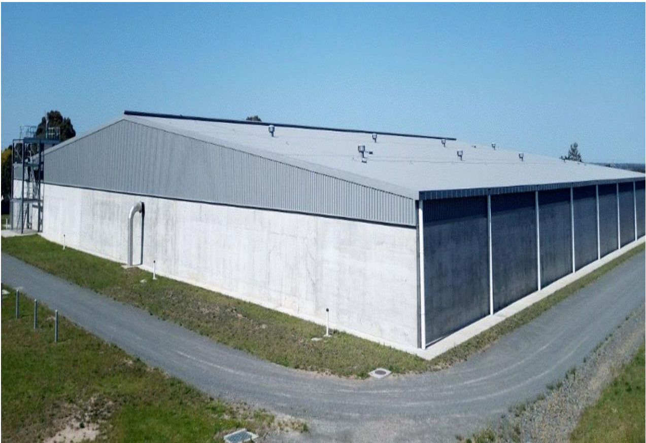
Photo: Re-commissioning the Wy Yung tank in preparation for summer.
